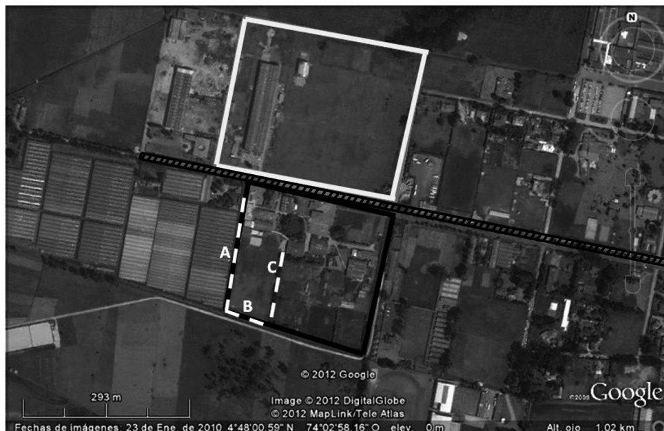
Fig. 1. University of Applied and Environmental Sciences, Bogotá, Colombia. A street divides the University in the two campuses (black dotted line). The northern campus (white box) is part of the Thomas van der Hammen Reserve, whereas the southern campus is in the city's urban expansion area (black box). Punctuated, white lines: sections where we evaluated the use of microhabitat and food selection (section B) and the use of space by the opossums (sections A, B and C). Image downloaded from DigitalGlobe © 2012.
