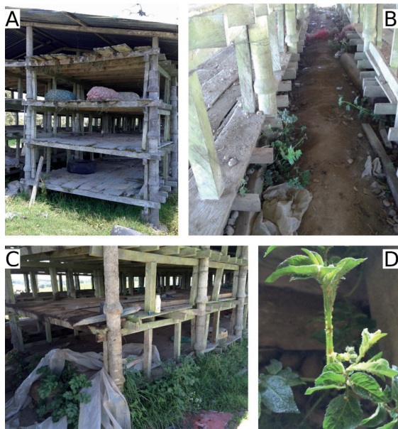
Figure 1. Condition of the rustic tuber-seed storage silo at Llanos de Cuivá (Yarumal, Antioquia) (A, B, C) where the volunteer potato plant used in this study was collected. A detail of the plant used in this study showing a high infestation by aphids (D).
