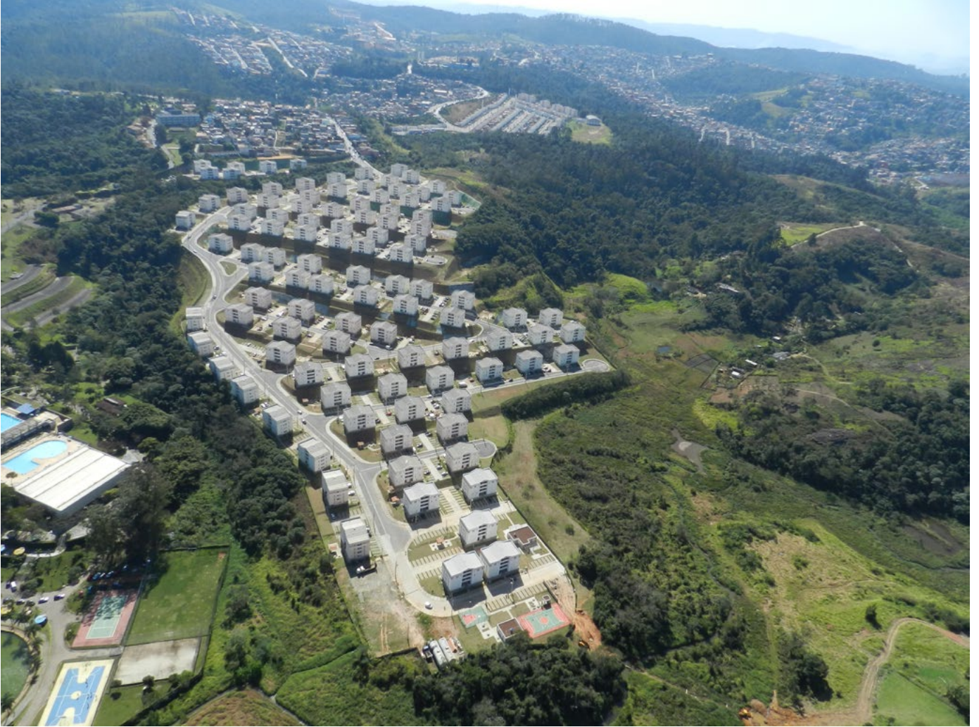
Image 4. Housing complex in Heliópolis slum. Architect: Hector Vigliecca
