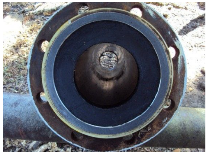
Figure 6. Test spool inspected without defects after 12 months in service
