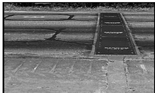
**Figure 3.** WIM system of flexible bands [35]
