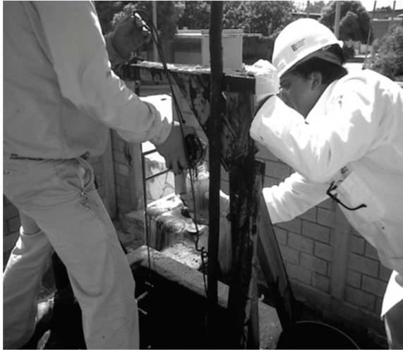
Figure 4. Injection plant, Tamaulipas-Constituciones field.
