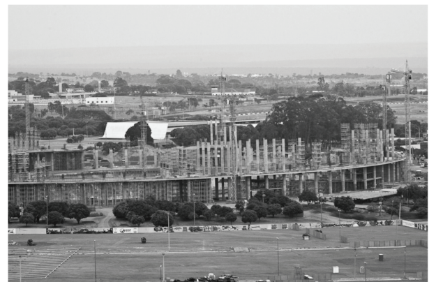
Figure 8. Picture from the recently finished sports arena in Brasilia during construction stage
