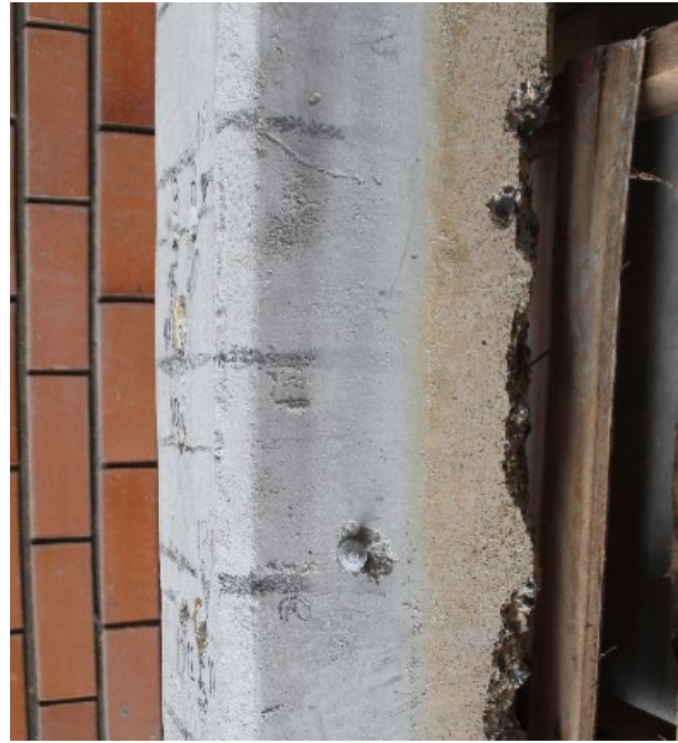
Figure 6. Surface of reinforced concrete column Source: Authors
