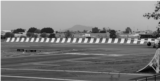
Figure 21. Curved deflector calculated and installed on five-left runway of the AICM. Source: Captured by authors on site.
