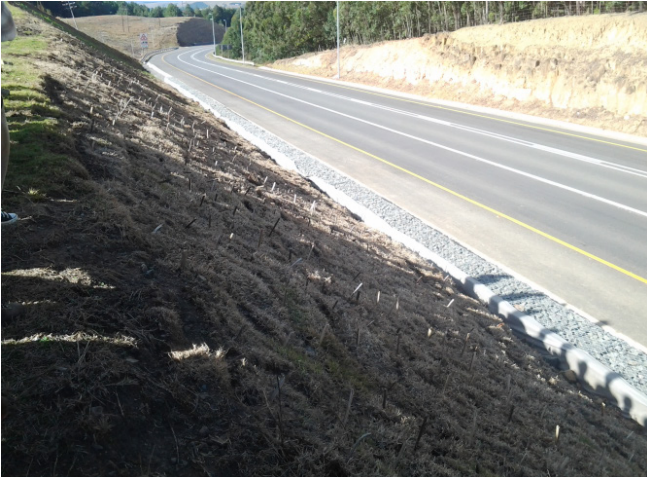
Figure 2. (a) Successful application of vegetation cover to control erosion on a roadside slope and (b) signs of erosion on a roadside slope due to the absence of vegetation cover.
