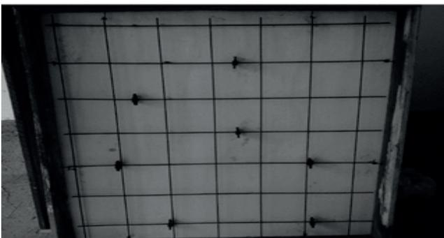
**Figure 5.** Reinforcement prepared inside the form before casting.
