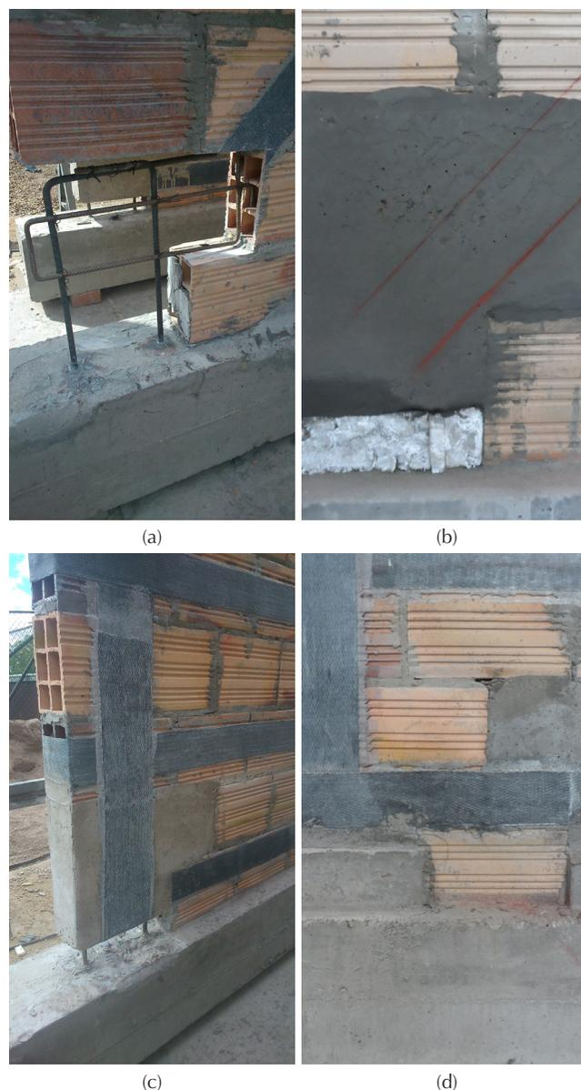
**Figure 3.** Construction process of the anchorage system: (a) removed masonry units and hooked steel bars; (b) placed grout block with bottom gap; (c) installed FRP strip wrapped around grout block; and (d) additional grout filling the gap.
