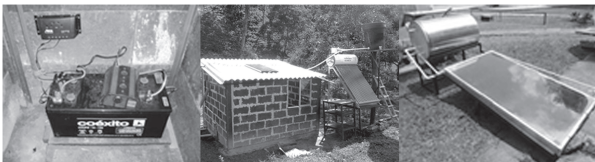
Figure 8. General and Final lay-out of the sustainable module housing: solar collector with vacuum tubes for 150 L, Photovoltaic System for 600Wh/day (20 A charge controller; 400 W Power Inverter; 100 Ah battery) and flat plate solar collector
