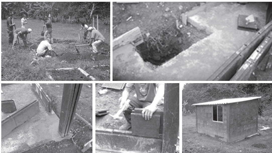
Figure 4. Ground Preparation, concrete base and columns foundations. Bricks and Columns Assembly. Finished Module.
