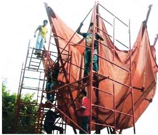
← Figures 79 to 87. Second deployment of the folding umbrella with membrane; in this second attempt, the regulators were open and this helped the membrane to be fully tensed. The project was a success. Source: Morales-Guzmán (2013).
