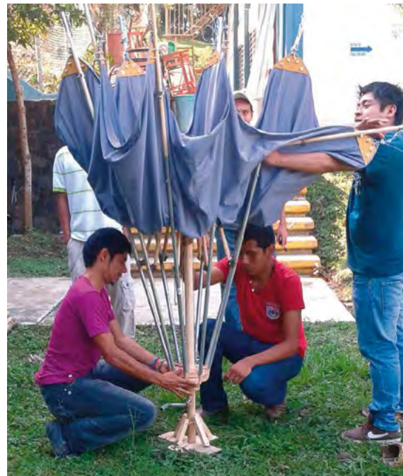
Figures 8 and 9. The unfolding of the model helped to form constructive concepts of the movement of the folding system of the umbrella.
