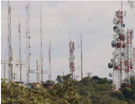
Fig. 3. Visual pollution caused by telecommunications infrastructure.
