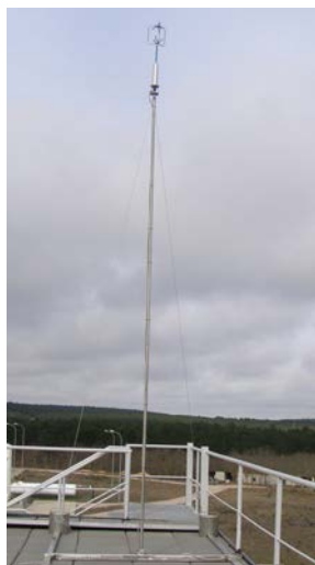
Figure 6 Meteorological mast for Enair EPRO70 Wind Turbine
