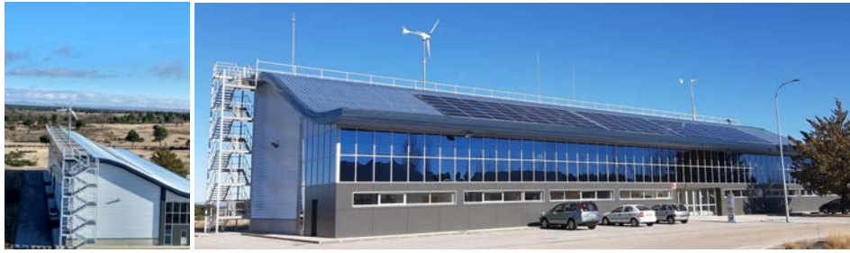
Figure 1 Enair EPRO70 Wind Turbine on the roof of LECA building
