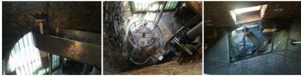
Figure 1 House of Silk lower gallery, with pico-hydro turbines, seen from the upper floor (auditorium)
