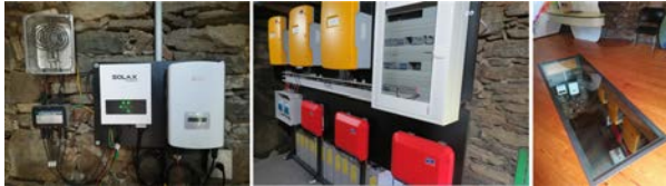
Figure 2 House of Silk upper gallery with microgrid (view from the upper floor at right)
