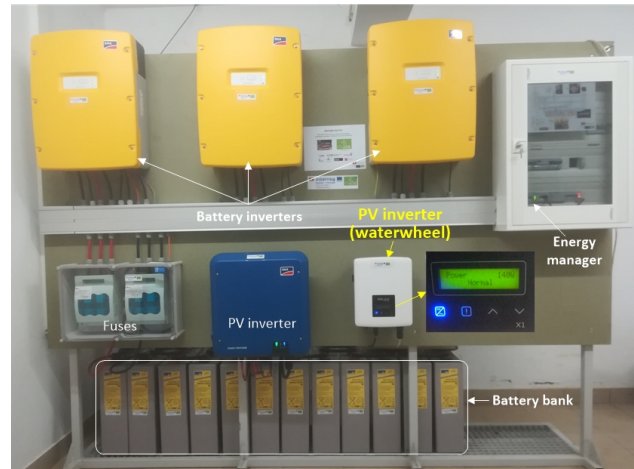
Figure 12 Smart microgrid installed in Castrelos' Aquaculture Centre
