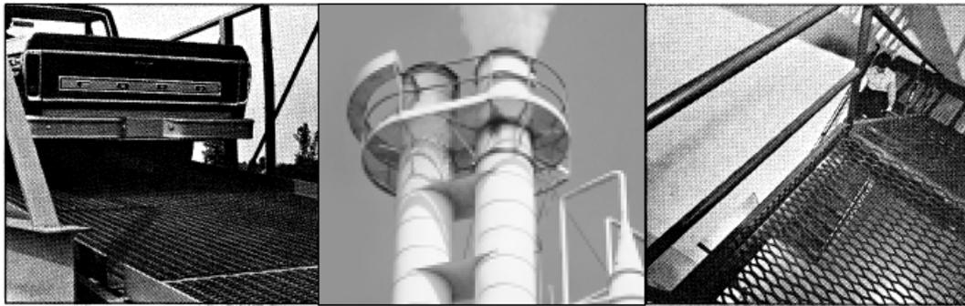
Figure 2 Applications of expanded metal meshes in support structures
