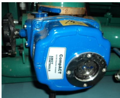
Figure 2 Thermostatic valve to control aftercooler temperature (Source: Porto do Pecem)
