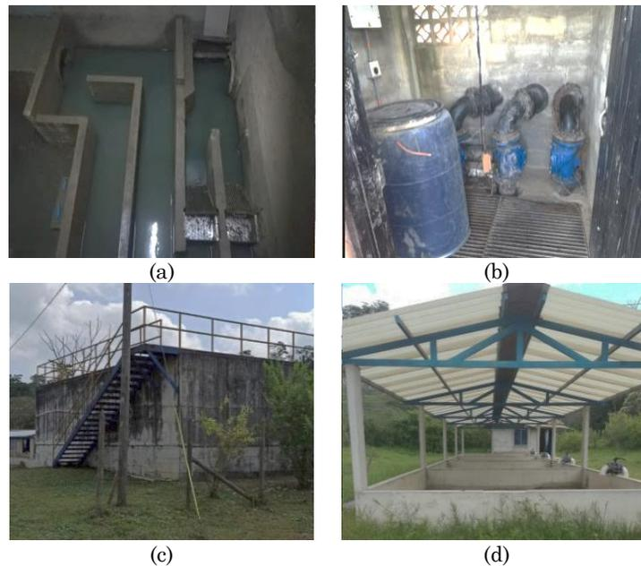
**Figure 4.** Treatment units in San Roque municipality WWTP. **a)** Preliminary treatment. **b)** Pumping station. **c)** UASB reactor. **d)** Drying beds. Source: Created by the authors.
